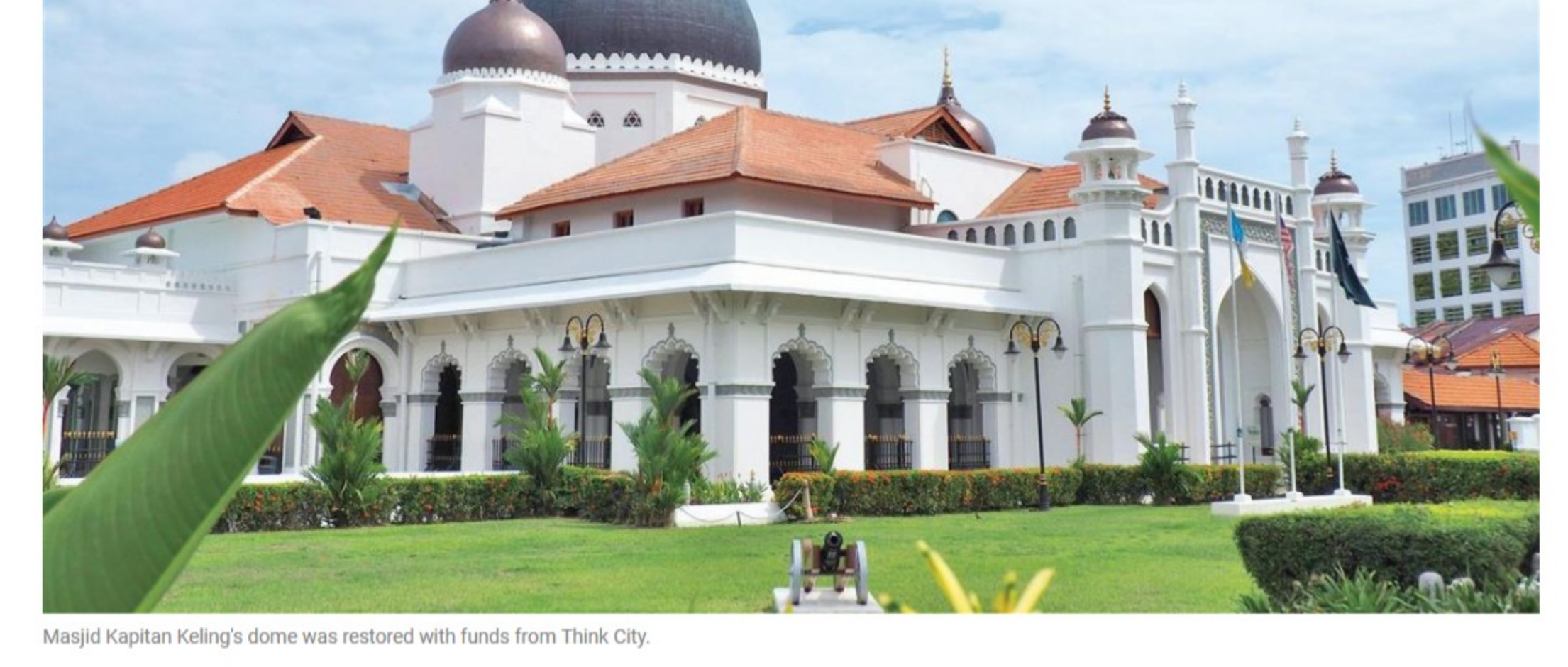
Masjid Kapitan Keling's dome was restored with funds from Think City.
